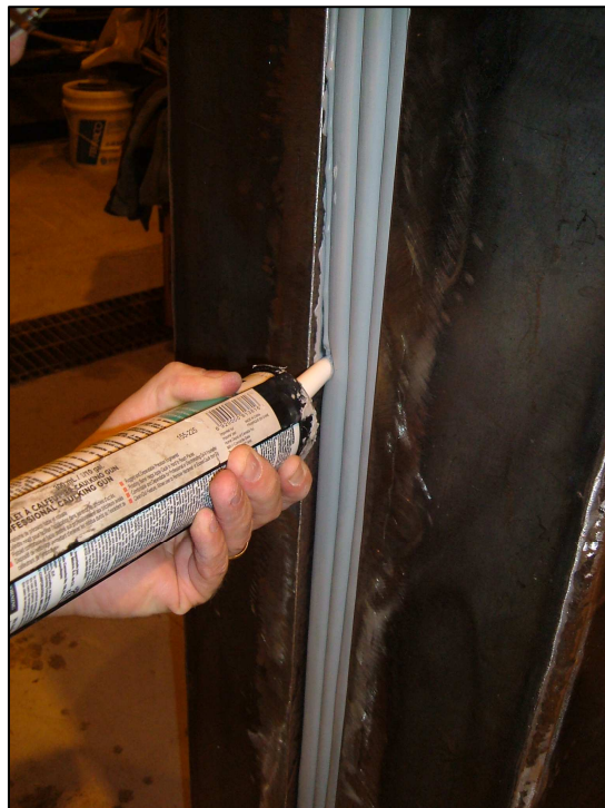
Figure A5 – Application of Dow Corning 790
